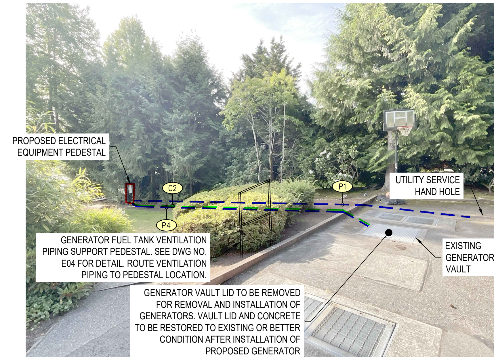
LIFT STATION 23 SITE NO SCALE
